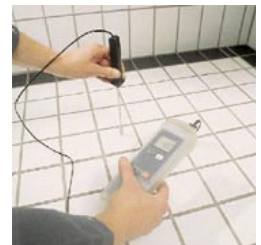
Checks floor heating
